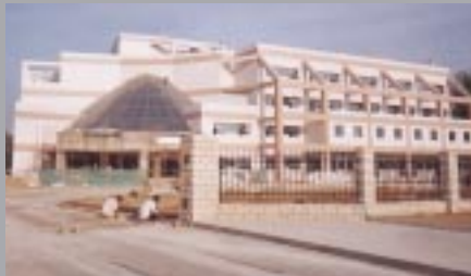
The Office Building of Curing Centre of Fourth ring Road in Beijing, China
